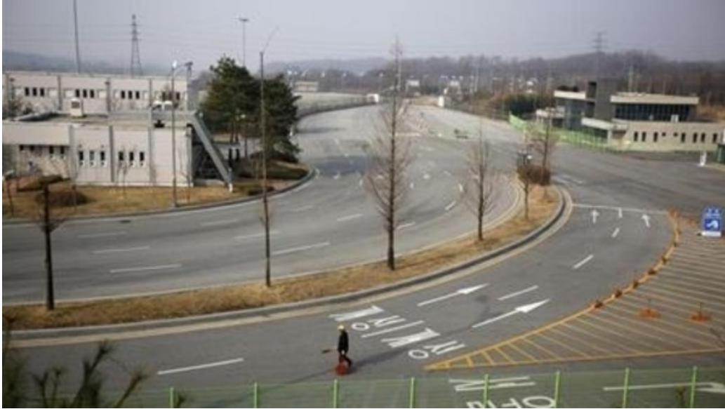
View of the now nearly deserted Kaesong Industrial Complex [Photo: Arirang News ]
