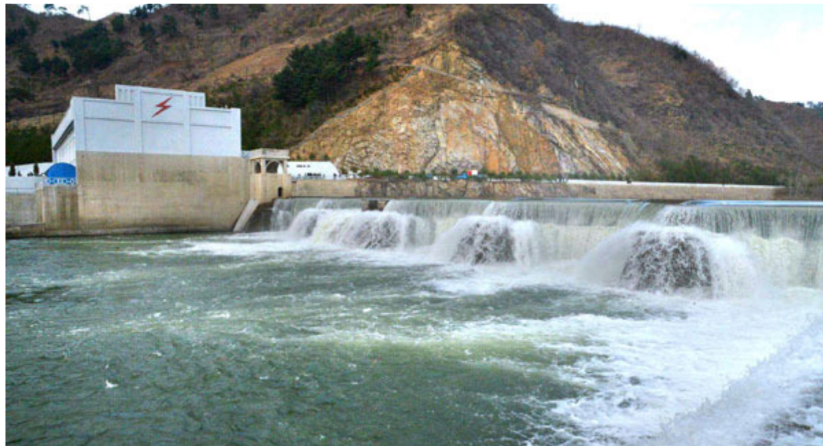
View of the newly operational Manpo Yonha Power Station [Photo: KCNA]
